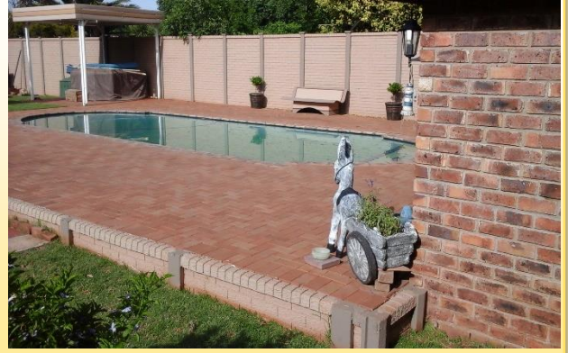
Low Retaining Wall
